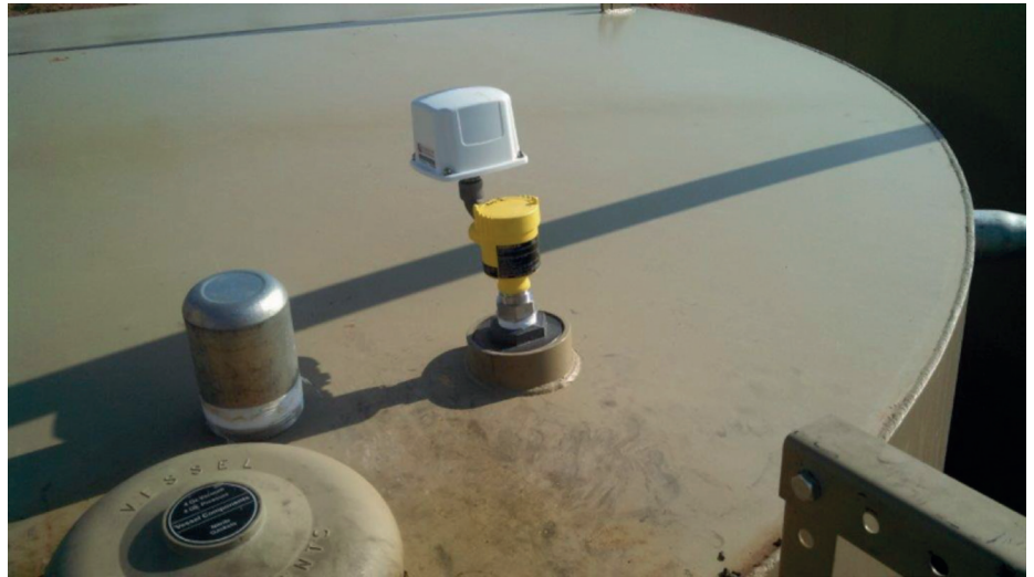
A SignalFire Sentinel HART wireless node connected to a guided wave radar sensor for tank level monitoring
