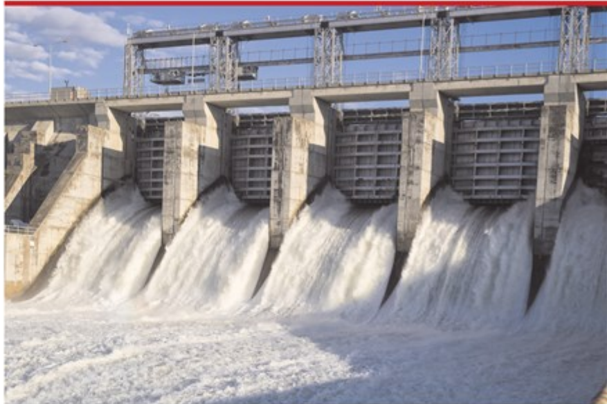
Traditional hard-wired monitoring systems can create reliability and cost challenges for operators, leading to increased interest in wireless options. Photo courtesy SignalFire Wireless Telemetry
